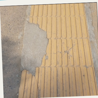
Can be Installed only on chipped surface
