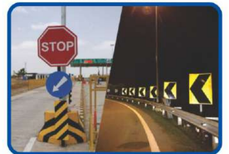
HAZARD MARKER AND CHEVRON SIGN BOARD
