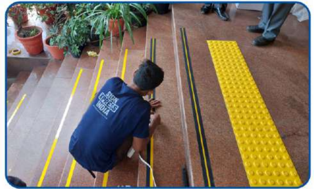
DSIIDC HEAD OFFICE
