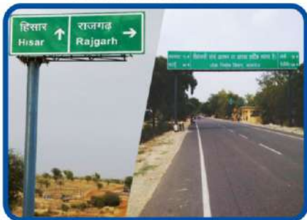
OVERHEAD GANTRY AND CANTILEVER SIGN BOARD
